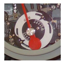
WTI Close up - showing alarm / trip - Figure 7a.
